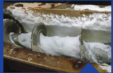
Salt build up inside a screw conveyor
